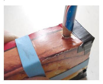
It should be just too small to insert the wooden dowel. Then take the wooden dowel and starting at an angle, rotate the dowel, enlarging the hole until it goes through. Make sure it has gone through both the front and back of the camera completely. Do this somewhat gently to avoid tearing the cardboard. There will be a burr of paper on the inside. Just leave it. It will help to prevent light getting into the camera.
